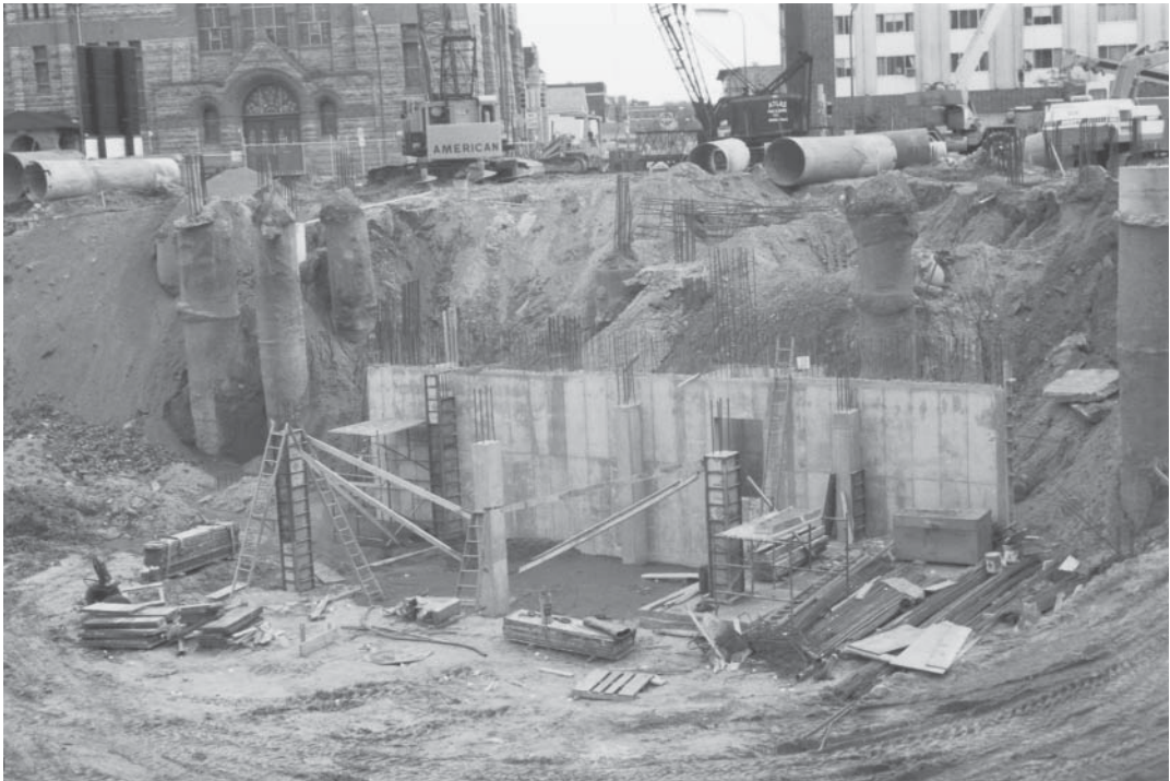
Wall and column footings, partly covered.
