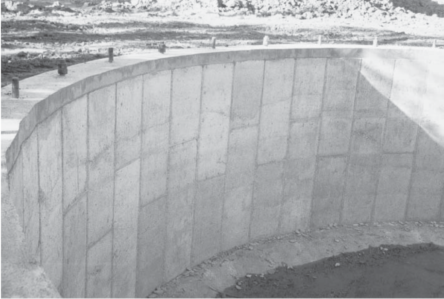
Reinforced concrete retaining wall.
