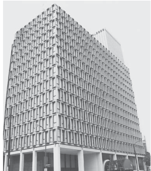
Office building, Chicago, Illinois.
