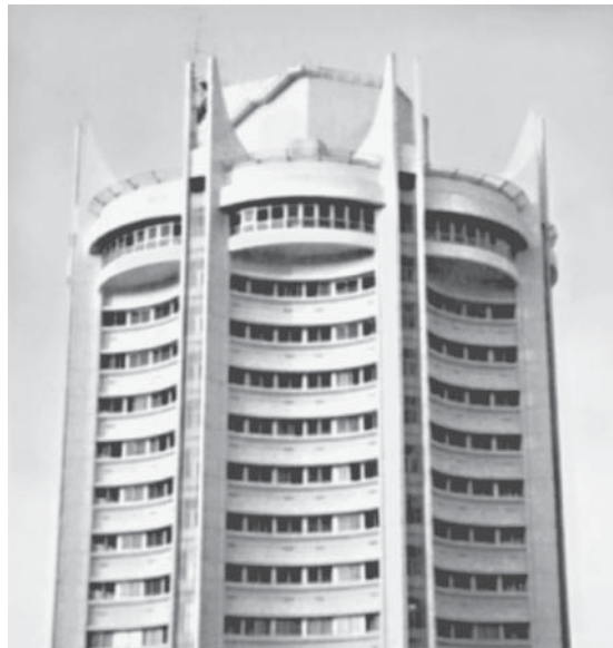
Circular beams in an office building.
