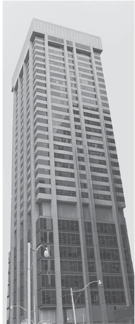
Columns in a high-rise building.
