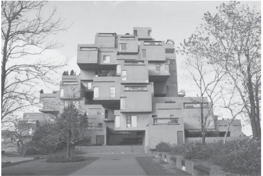
Apartment building, Habitat 67, Montreal, Canada.
