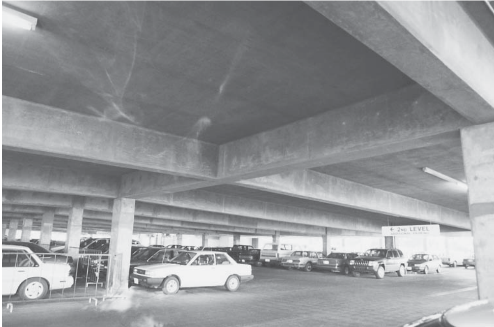
Slab on beams.
