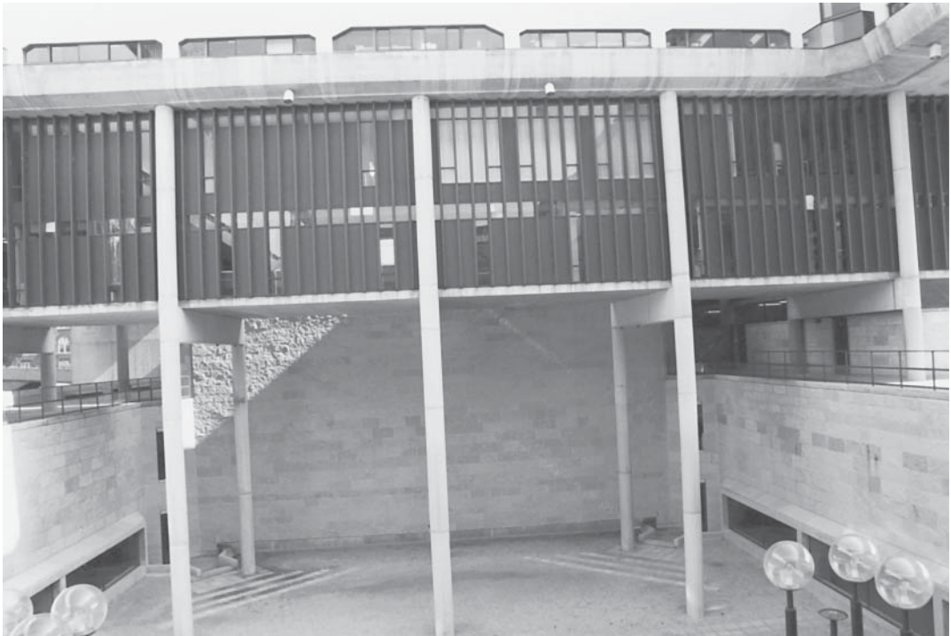
Columns, University of Wisconsin, Madison, Wisconsin.
