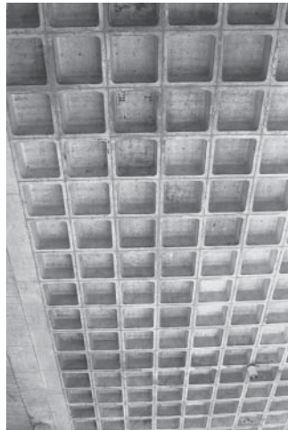
Waffle slab (looking upward).
