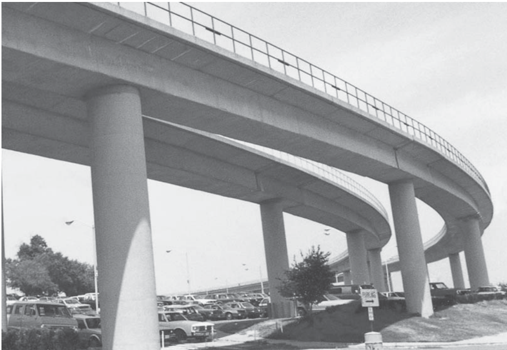
Curved-beam bridge, Washington, D.C.
