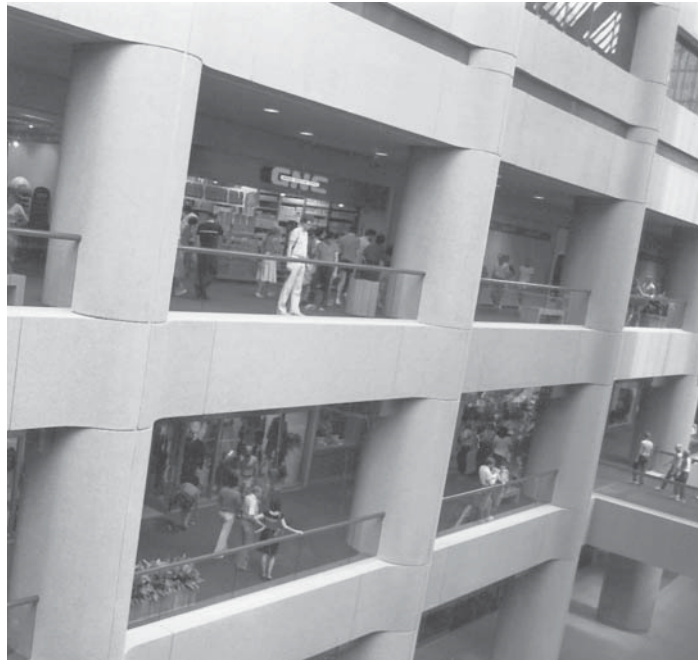
Columns supporting 52-story building, Minneapolis, Minnesota. (Columns are 96 \times 64 in. with round ends.).
