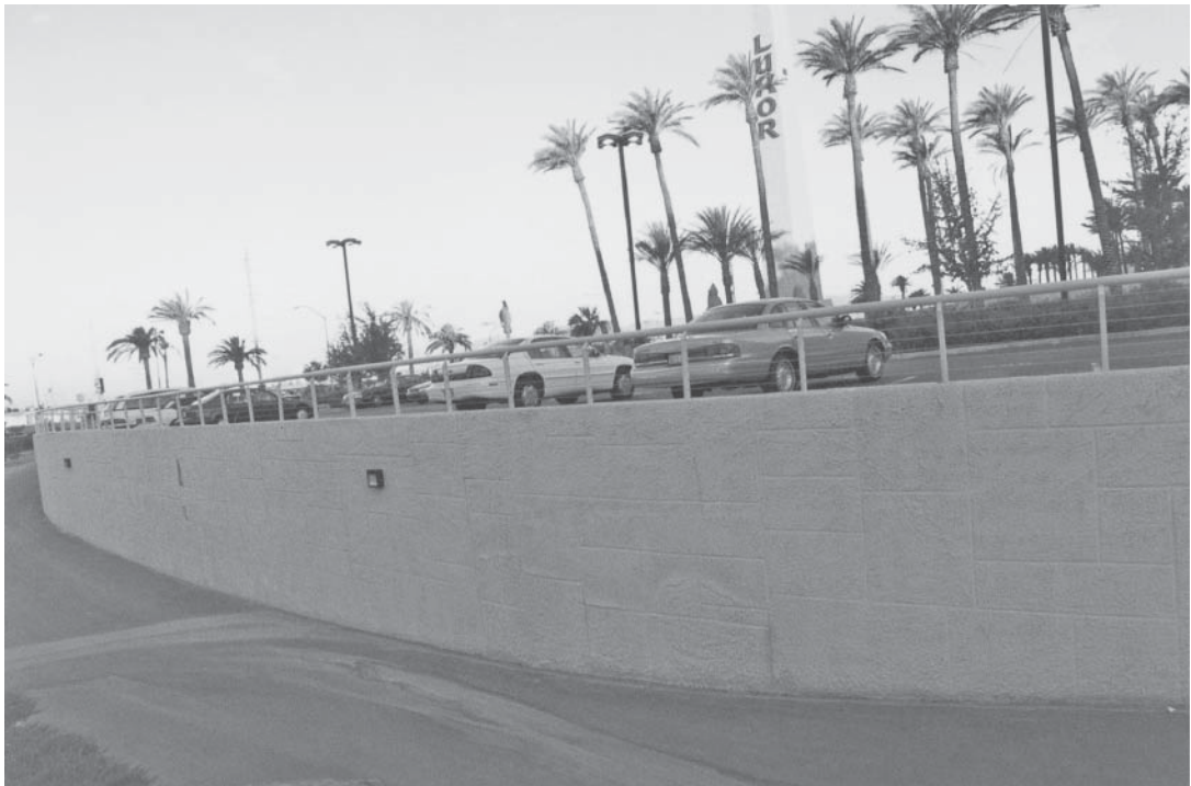
Retaining wall in a parking area.
