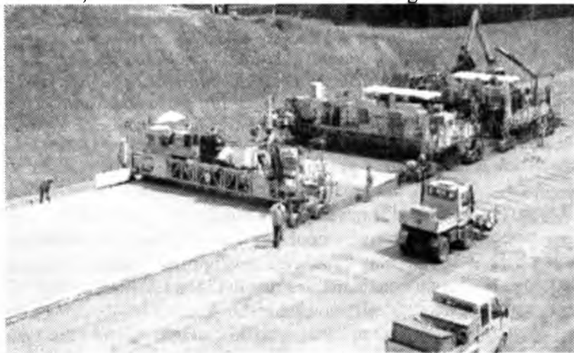
4.10-rasm. "Wirtgen" firmasining SP-1500 modelidagi betonyotqizgichi
