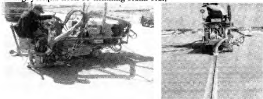
4.30-rasm. Ko‘ndalang va bo‘ylama choklarning ochilishi
