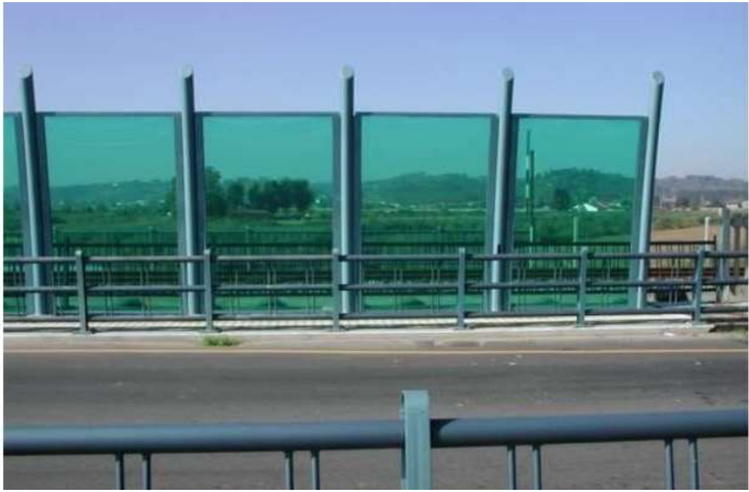
12-rasm. shishali polysorbonat materialidan to'siq
