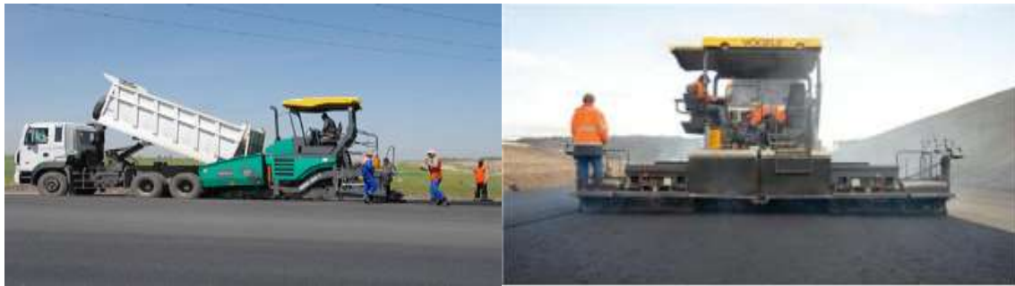
19-rasm. Issiq asfaltobeton qarishmasini yo‘lga yotqizish texnologik jarayonida lavxalar.
