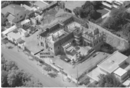
Fig. 1. State of building before move
