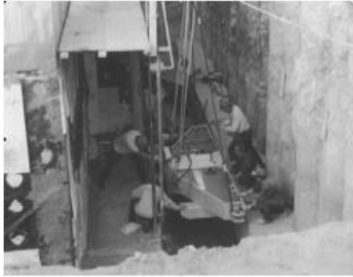
Fig. 8. Placement of hydraulic jacks
