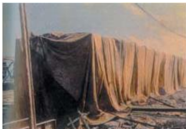
Beam under steam curing.
