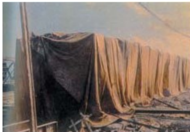
Beam under steam curing.
