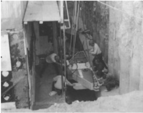
Fig. 8. Placement of hydraulic jacks
