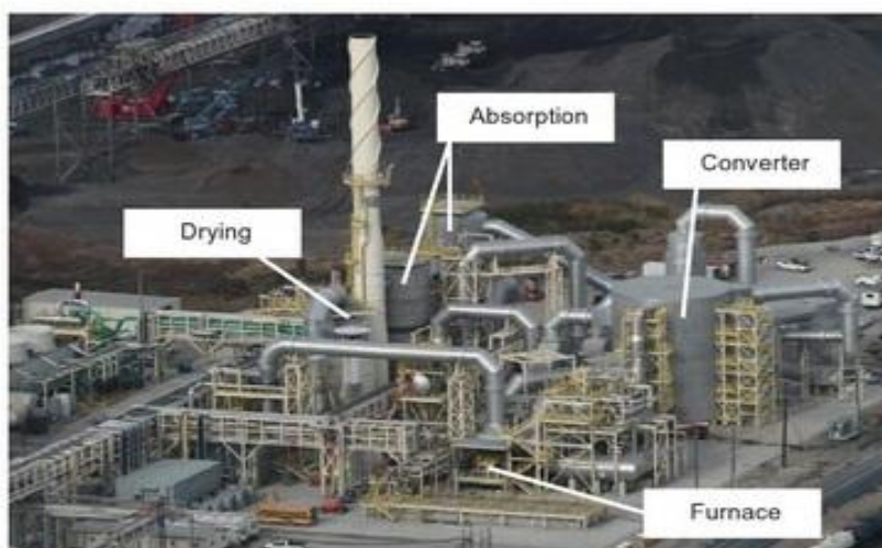
Figure 12 Modern 4100 tonnes/day sulfur burning sulfuric acid plant, courtesy PCS Phosphate Company, Inc. (2012). The main components are the catalytic \text{SO}_2 oxidation “converter” (tall, right), twin \text{H}_2\text{SO}_4(l) making (“absorption”) towers (middle, right of stack) and a sulfur burning furnace (middle, bottom). The air dehydration (“drying”) tower is left of the stack. The catalytic converter is 16.5 m diameter.
