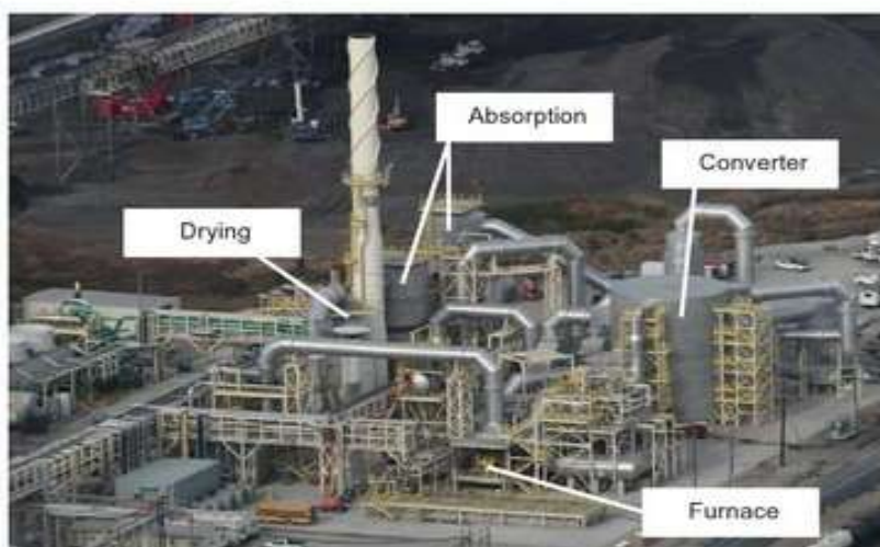
Figure 12 Modern 4100 tonnes/day sulfur burning sulfuric acid plant, courtesy PCS Phosphate Company, Inc. (2012). The main components are the catalytic SO 2 oxidation “converter” (tall, right), twin H 2 SO 4 (l) making (“absorption”) towers (middle, right of stack) and a sulfur burning furnace (middle, bottom). The air dehydration (“drying”) tower is left of the stack. The catalytic converter is 16.5 m diameter.
