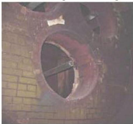
Figure 13 Burner end of sulfur burning furnace. Atomized molten sulfur droplets are injected into the furnace through steam-cooled lances. Dry combustion air is blown in through the circular openings behind. The sulfur is oxidized to \text{SO}_2 by Reactions (3.1) and (3.2). Atomization is done by spiral or right angle flow at the burner tip.
