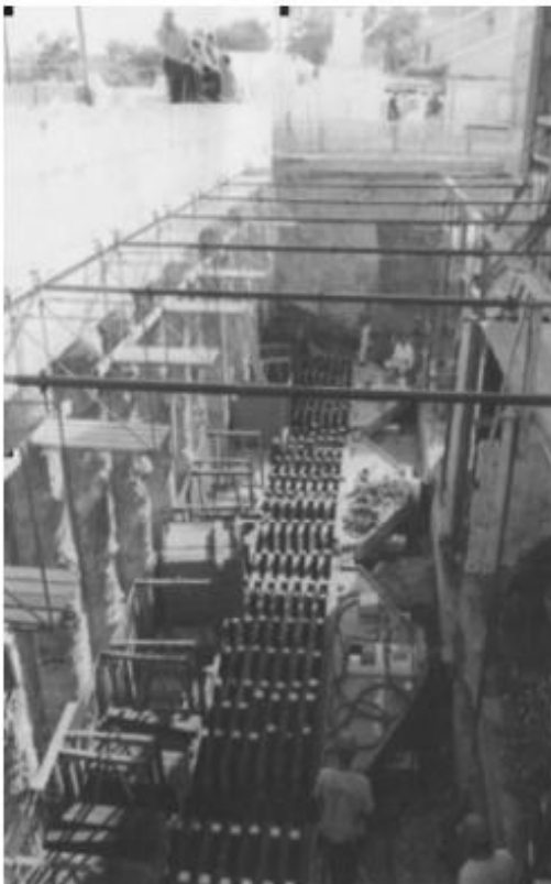
Fig. 9. Push in progress and timber cribbing being used
