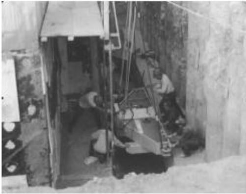
Fig. 8. Placement of hydraulic jacks
