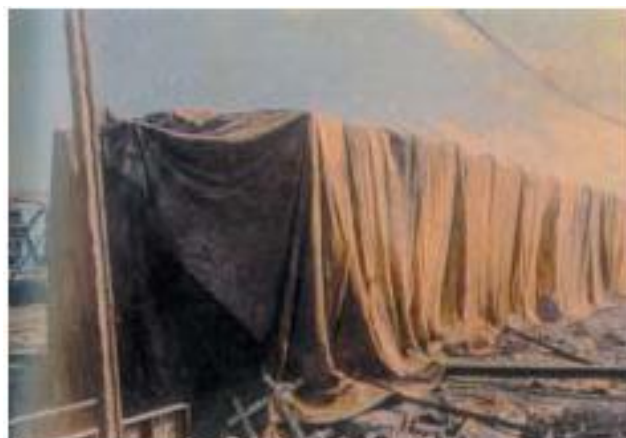
Beam under steam curing.
