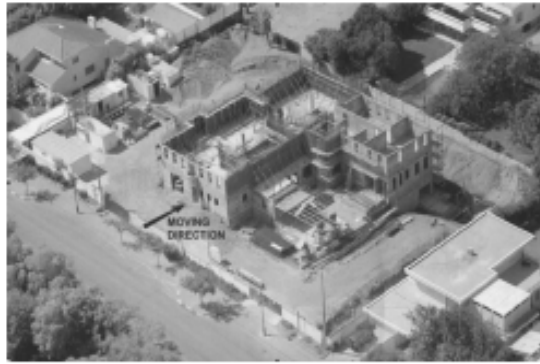
Fig. 1. State of building before move
