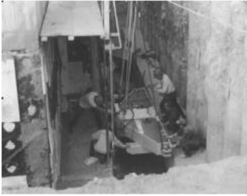
Fig. 8. Placement of hydraulic jacks
