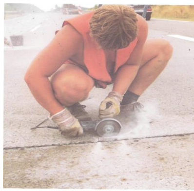
4.17-rasm. Sementbeton choklariga qo'lda ishlov berish
