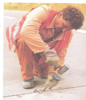
4.17-rasm. Sementbeton choklariga qo'lda ishlov berish
