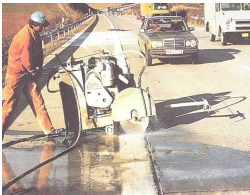
4.16-rasm. Maxsus mashinada sementbeton choklariga ishlov berish
