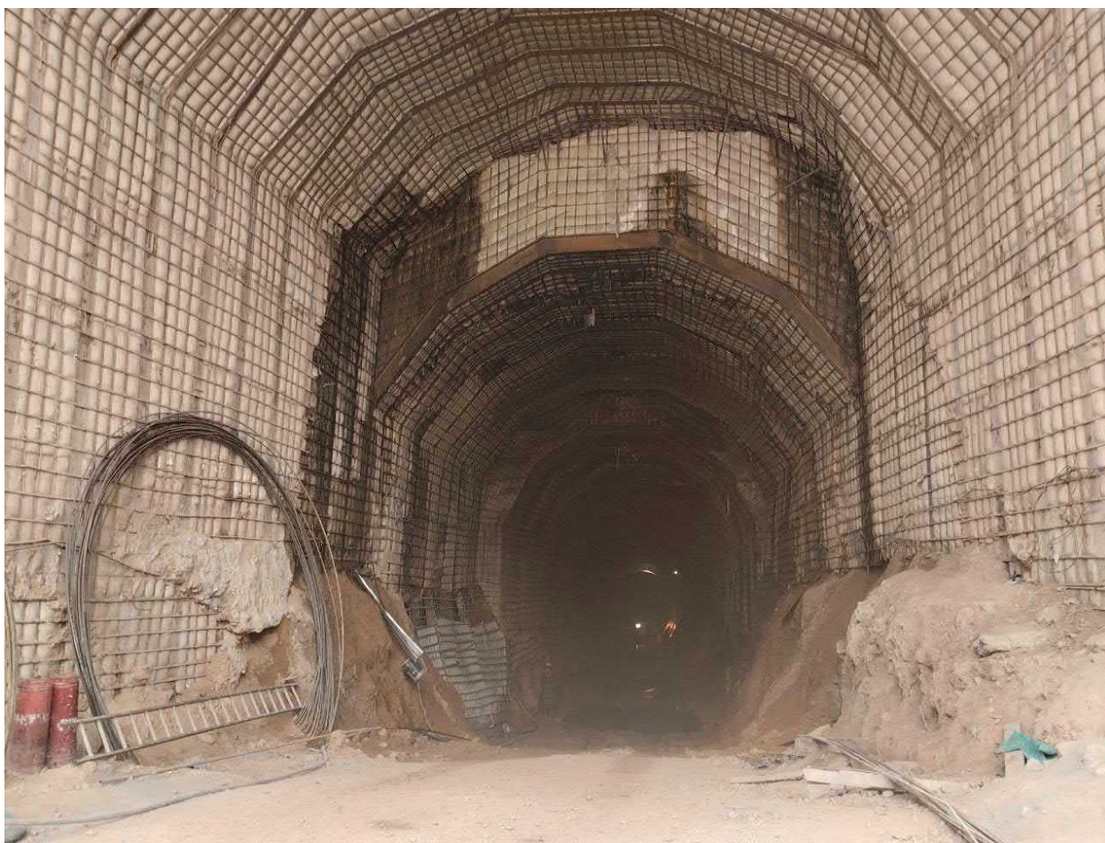
2.5 – rasm. Temirbeton bilan mustaxkamlangan tunnel kirish qismi.
