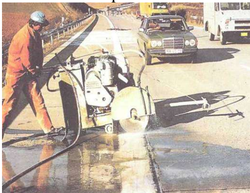
5.16-rasm. Maxsus mashinada sementbeton choklariga ishlov berish
