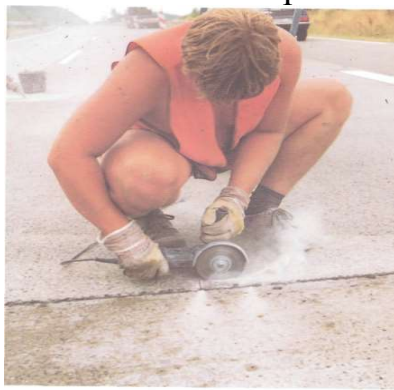
5.17-rasm. Sementbeton choklariga qo'lda ishlov berish
