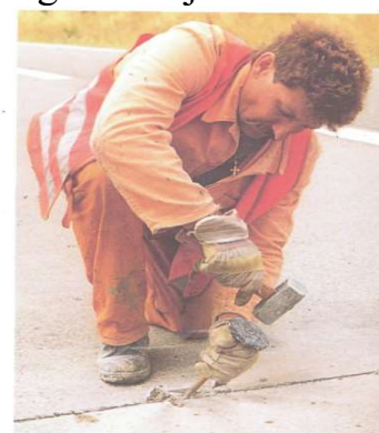
5.17-rasm. Sementbeton choklariga qo'lda ishlov berish
