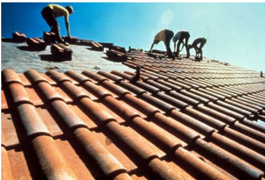
4- rasm. Plitkalarni yotqizish.
