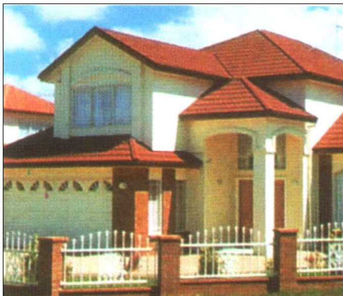
3.11-rasm. Metrobond bilan qoplangan tom
