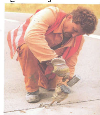
5.17-rasm. Sementbeton choklariga qo'lda ishlov berish
