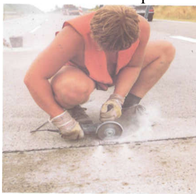
5.17-rasm. Sementbeton choklariga qo'lda ishlov berish
