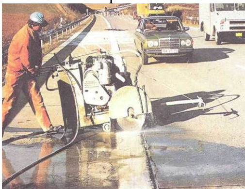
5.16-rasm. Maxsus mashinada sementbeton choklariga ishlov berish
