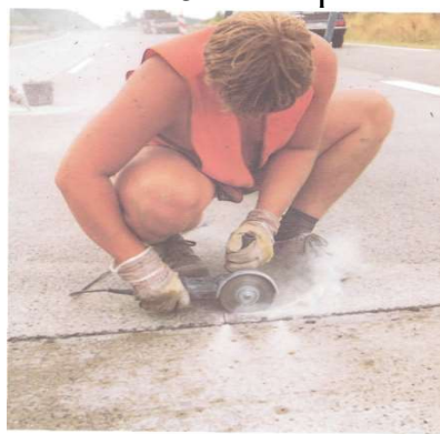
5.17-rasm. Sementbeton choklariga qo'lda ishlov berish
