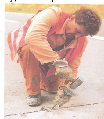
5.17-rasm. Sementbeton choklariga qo'lda ishlov berish
