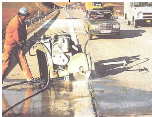
5.16-rasm. Maxsus mashinada sementbeton choklariga ishlov berish
